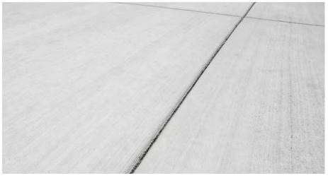
Fig.68 Example of broom finish concrete paving
