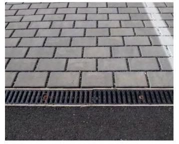
Fig.80 Permeable paving in a parking lot
