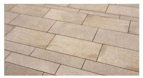
Fig.69 Example of drivable pavers
