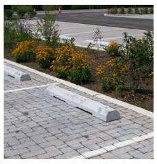
Fig.54 Permeable paving in parking lot
