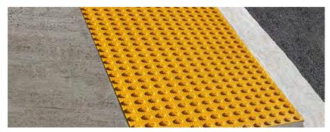
Fig.40 Tactile paving for visually impaired users
