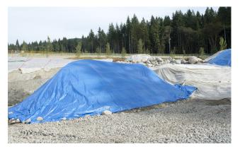
The placement of polyethylene tarps must be completed such that the overlapping margins of the tarps is folded and secured to prevent disturbance by wind. An effective measure to secure tarps is the anchoring of overlapping seams with a length of plastic snow fencing anchored with landscape staples installed at 0.5m centers along the plastic seam.
