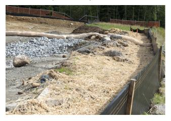
Silt fencing should not be installed on steep slopes (e.g. ≥2H:1V), rather fencing should be installed approximately 1m below or beyond the toe of slope inflection to provide appropriate sediment retention capacity. Sediment accumulations exceeding 1/3 of the fabric height must be removed.
