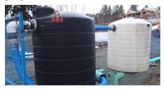
Portable tanks may also provide suitable detention in support of localized dewatering requirements where discharge to the municipal storm system or watercourses would be prohibited due to turbidity levels.
