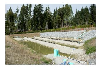
Sediment control ponds should include a pre-treatment sump to facilitate the deposition of the largest sediments in transport. The pre-treatment sump should be a minimum 0.5m deeper than the remaining pond invert, and be separated by 3" fractured rock berm set a minimum of 0.5m above the normal pond invert. The pre-treatment fore-bay should include measures to facilitate clean-out of deposited materials as required.
