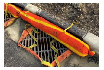
2. Sediment Barrier Berms/Check Dams – Berms or check dams in the context of inlet protection refer to the installation of temporary barriers installed in conjunction with filter sock inserts to augment the intended function of the inlet protection measures. Berms may consist of rock mulch, fiber rolls, or straw wattles installed along the rear openings of storm inlets to preclude the bypass of sediment laden runoff past filter sock inserts.
